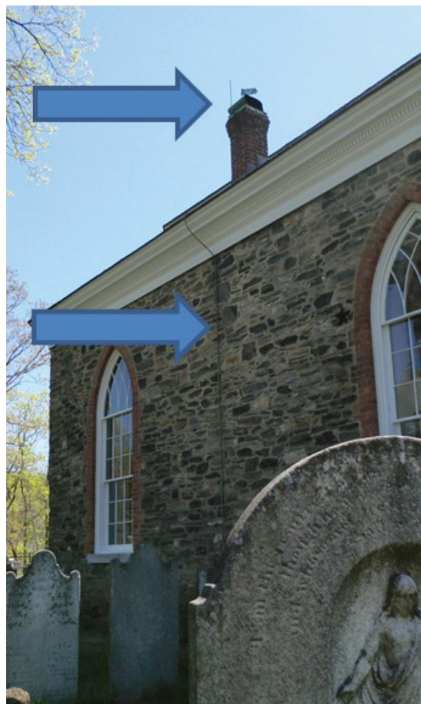
Figure TF2-2: Lightning rod and grounding cable on Old Rock Church at Sleepy Hollow, New York. The lightning rod attracts the strike by concentrating charges at its tip. The cable shunts the current to ground, carrying it on the outside of the (rock) church, rather than on the inside where materials (wood, plaster, etc.) are more flammable. The cable is large enough in diameter to carry the current without burning, although it will still be hot to the touch after a lightning strike.
