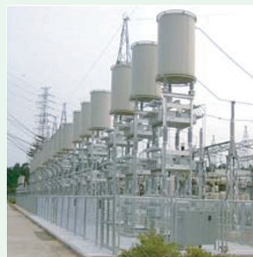
Figure TF26-2: A bank of large capacitors for three phase power. (Note the 3 lines going in and out of each capacitor.)
