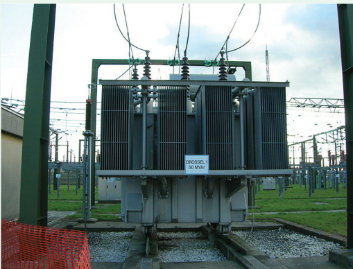
Figure TF26-1: A large 50 MVAR (Mega-Volts-Amps Reactive) loading inductor.
